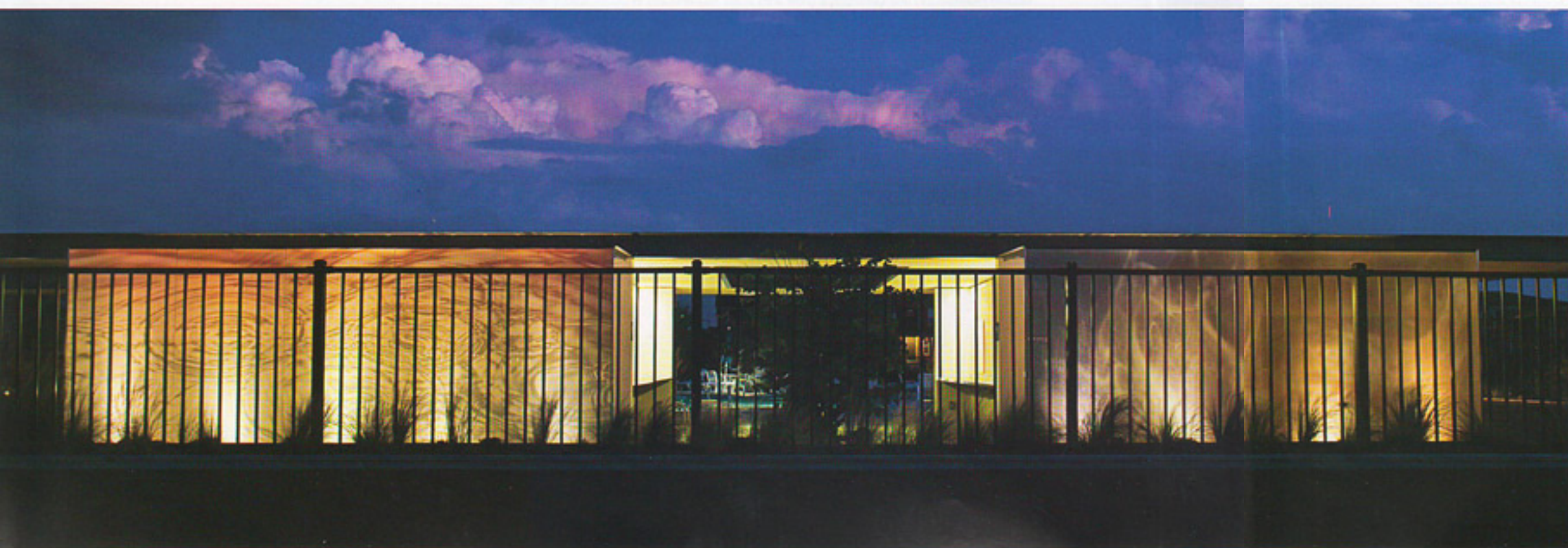
LEFT: A 150-foot planter box that stretches the length of the pool house was constructed out of reclaimed sheets of metal from the Stapleton International Airport.
